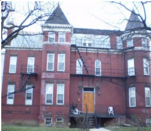
Oxford House - Nineteenth Street 1238 Harvard St NW Washington, DC 20009 10 M • March 1, 1982
